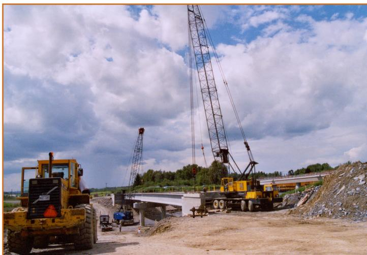
*Considerable damage and expense was incurred, and two highway construction workers were injured, during a complex tandem lift involving two cranes. A 90-foot lattice boom collapsed when the work radius and weight capacity of a crane to lift a 40-foot concrete beam was miscalculated. The cause of the incident was a failure to stay within the crane's safe operating limits.*
